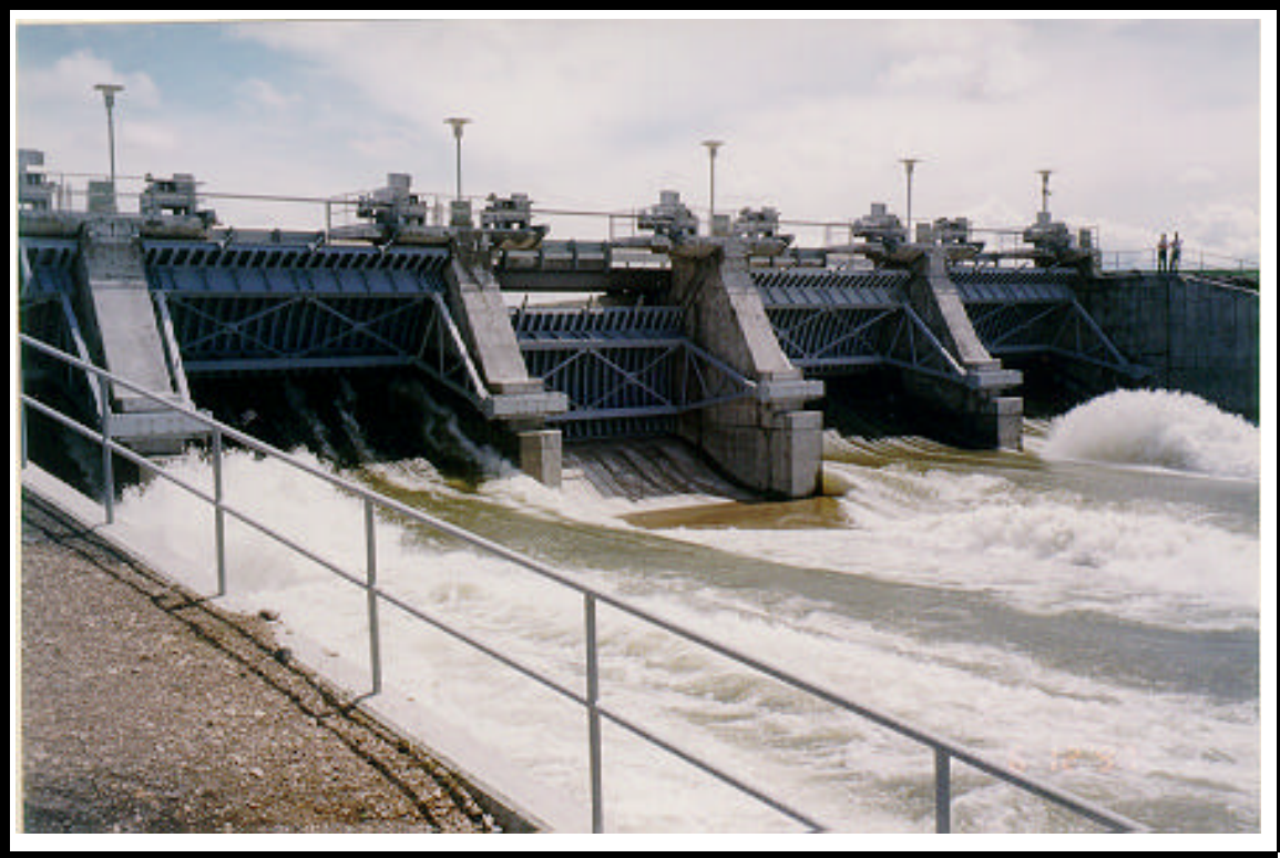
MilnerDam spillway discharge. Four of the five spillway gates are being used to pass the river flow in excess of the capacity of the three irrigation canals (Gooding, Northside, and Southside canals) and two powerhouses (at-site and downstream powerhouses) that are fed by this project.
