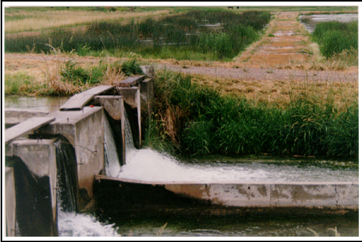
Cedar Draw Research Project. Irrigation return flow enters the raceways, now settling ponds, from the supply manifold, then to the rearing ponds (background upper right) where high nutrient-using plants consume the chemicals before the water is released back into the river. This is an energy efficient continuous gravity system.
