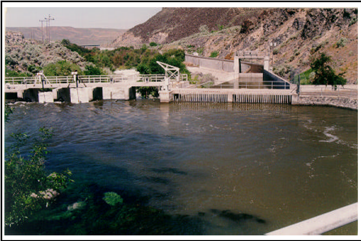
Lower Malad flume entrance. The entrance to the Lower Malad powerhouse flume is located in the Upper Malad afterbay. The flow into the flume is controlled by a flume gate and the river gate structure. Note that the flume gate is closed (powerplant is out of service), diverting the water back into the river. US 30 bridge is in the background.
