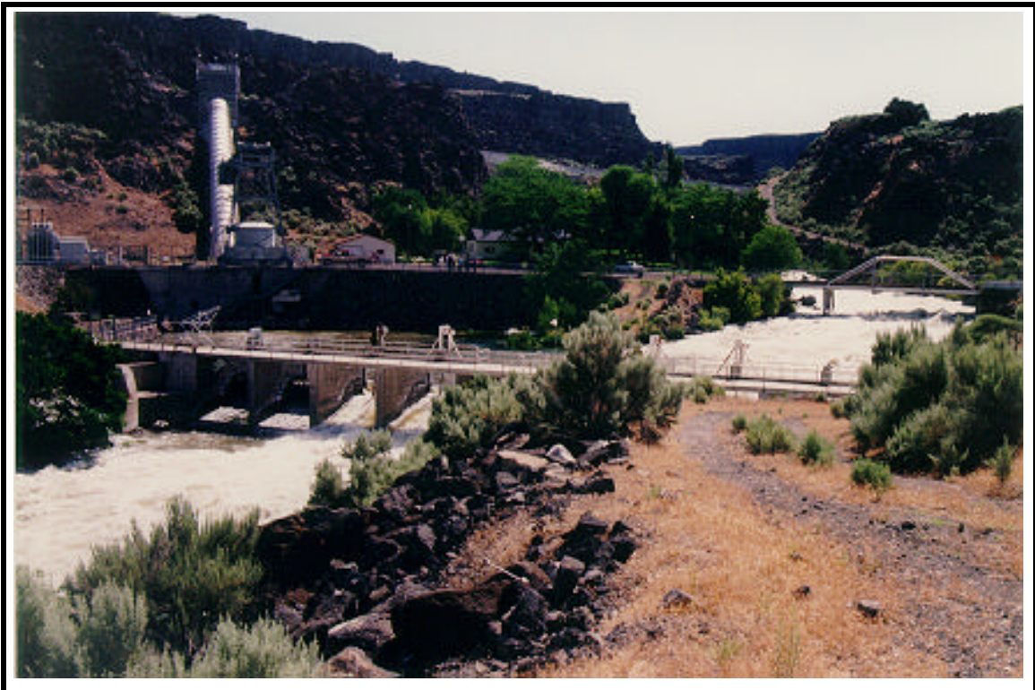
Upper Malad Powerplant. Penstock leads from flume to powerhouse. Typically all the river flow is diverted into the powerhouse flume. At this time the river flow exceeds flume capacity by an estimated 3000 cfs. Flow in the Lower Malad flume is partially controlled by diversion structure.
