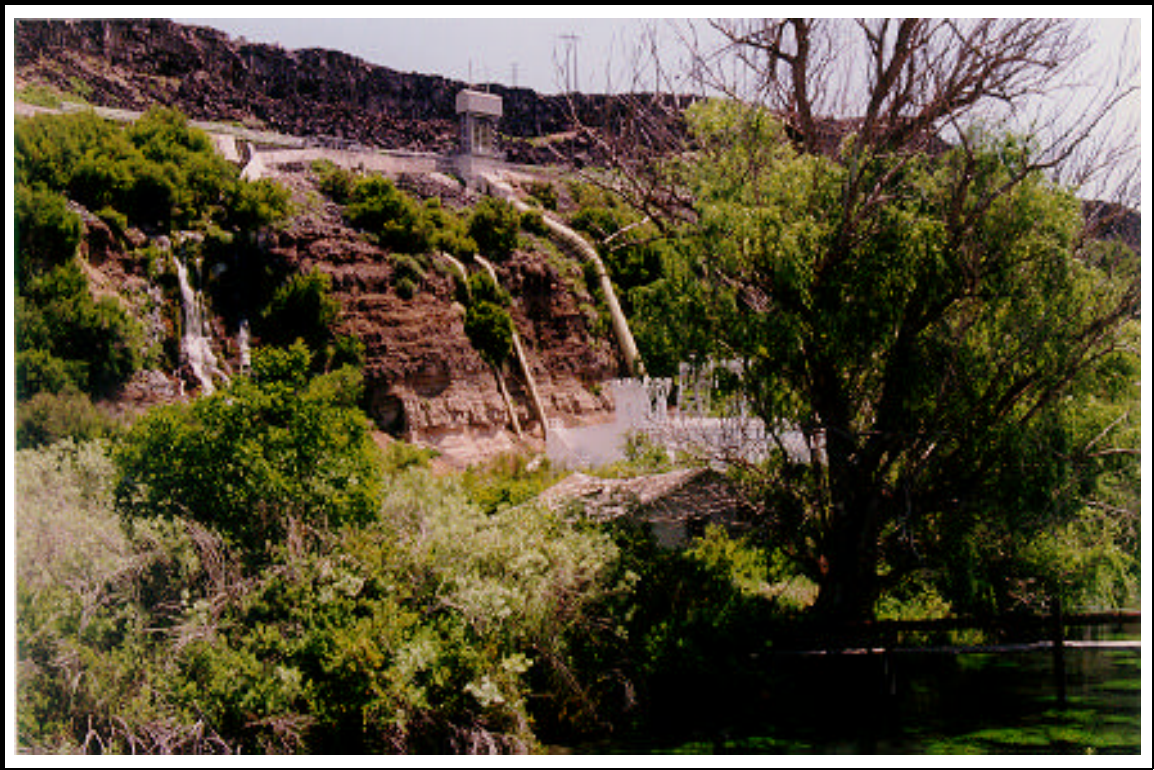
Thousand Springs Powerplant with collection flume and untapped springs to left of penstock. These springs are the outlet of the Lost River which disappears underground into the lava beds 100 miles to the northeast near Arco, Idaho. Note unique architectural style of powerhouse.
