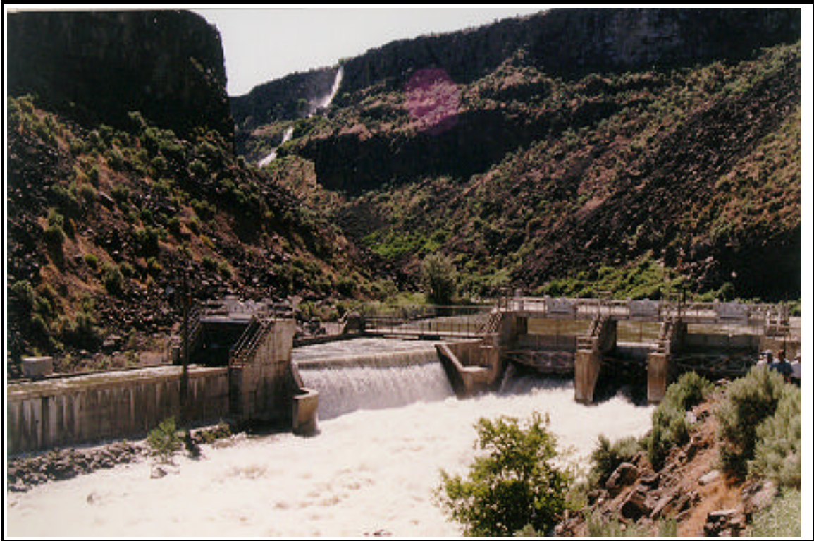
Upper Malad Powerplant flume diversion dam. River flow greater than the flume and powerhouse capacity is diverted back into the river channel. Both canal; overflow section and diversion dam gates are used to bypass excess flow. Note irrigation return flow coming off cliff.
