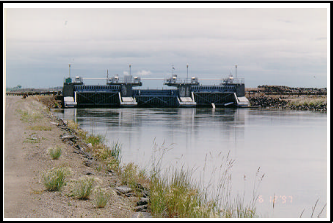
Control structure on southside canal (one mile below Milner) controls both the flow into the downstream powerhouse, which is located just upstream and to the left of this structure, and the irrigation flow in the canal.
