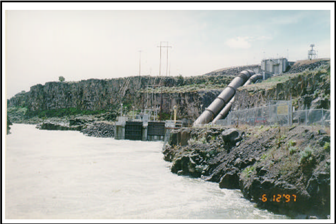
Milner Downstream Powerhouse. The Southside canal carries 8500 cfs from the Milner pool to feed the south side canal irrigators and the Milner downstream powerhouse, which has a capacity of 5.5 kcf and 58.5 MW from the two units. Powerhouse inflow is controlled by the structure pictured above.
