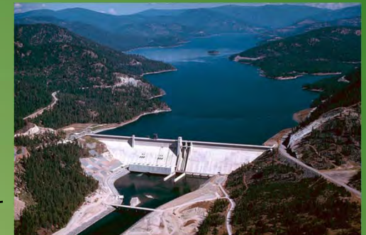
Libby Dam RM 222
