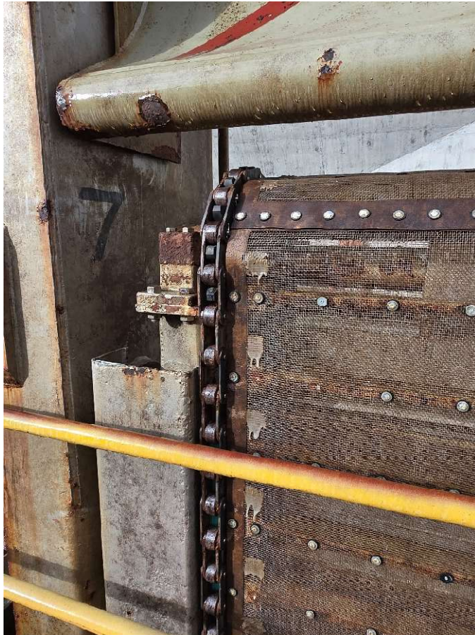
Figure 3: Photo of a representative existing screen at BON. BON and JDA are proposing to install new screen material in a few units this winter. New screen material has ~1" wider border strip on the edge (and does not have glue patches).
