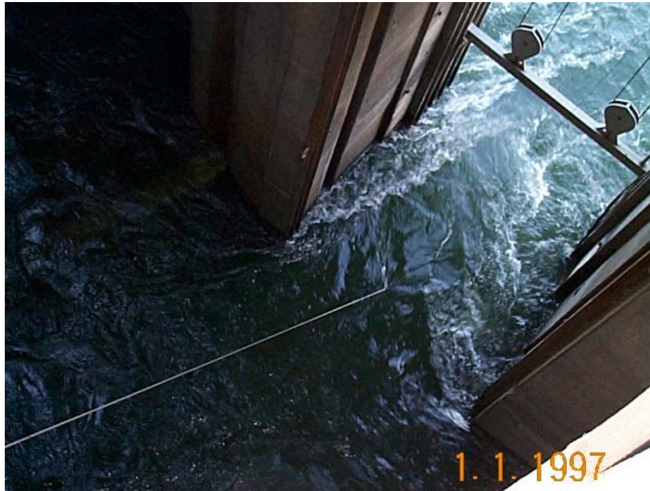
Figure 2: Photo of North Entrance Weir Gate WG-64
