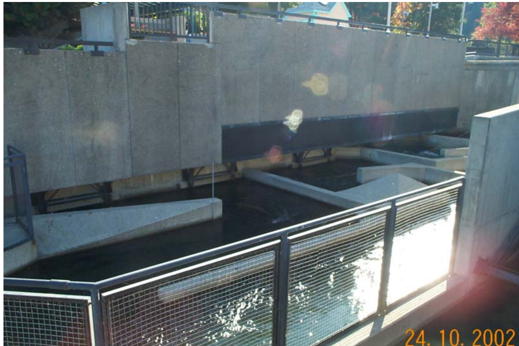
Figure 4: Counting Station, Counting Bypass Slot and Exit Channel
