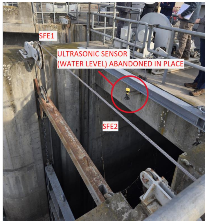
Figure 4: SFE1 & 2 Original Tailwater Sensor
