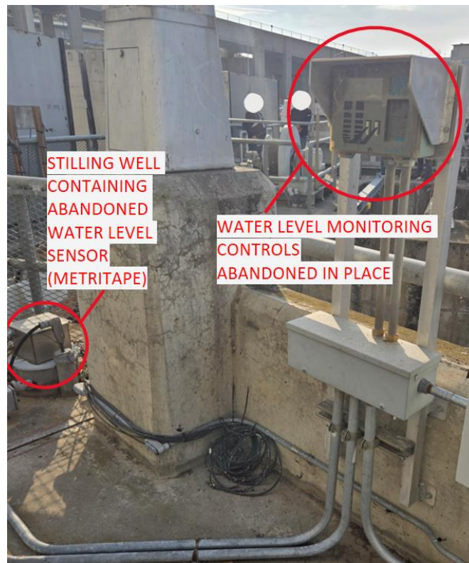
Figure 6: Stilling Well & Abandoned Devices
