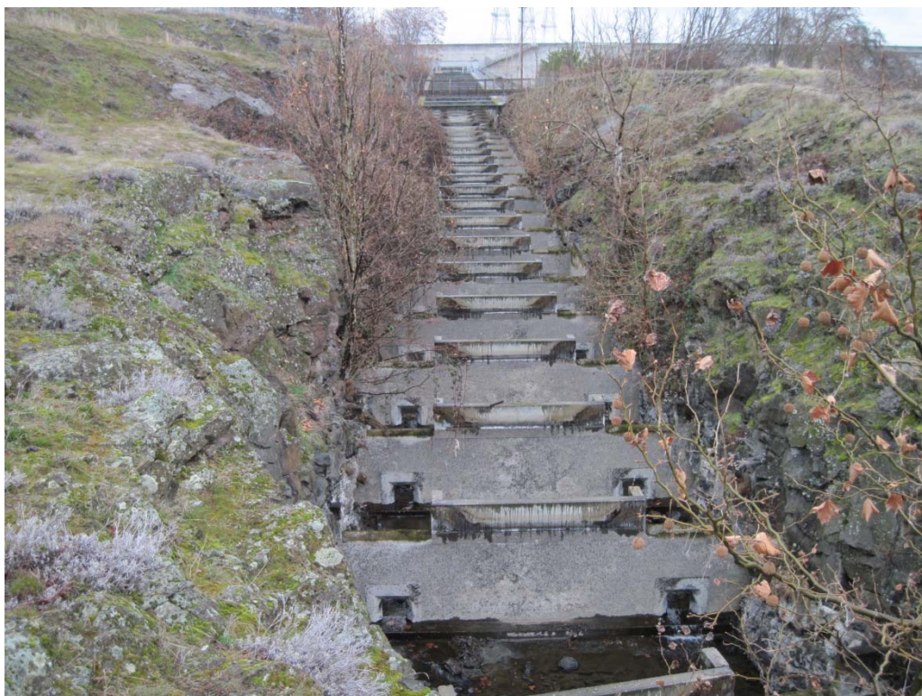
Photo 1 - looking north up fish ladder.
