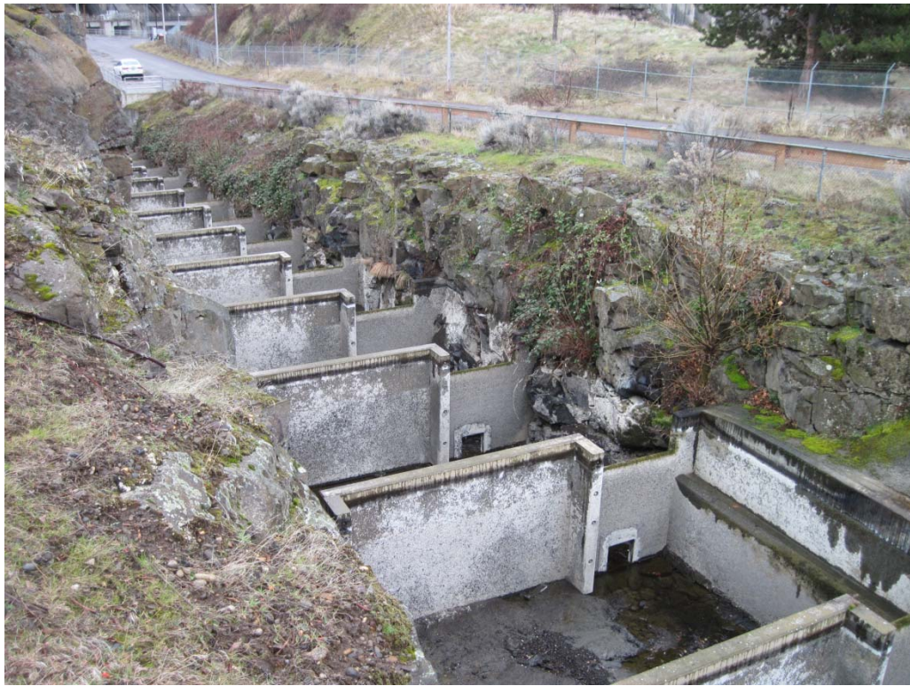
Photo 9 – Looking towards the southern section of the fish ladder.
