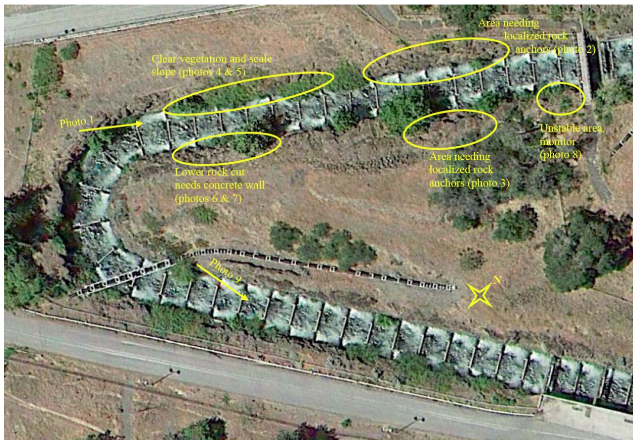
Figure 1 - Aerial photo showing north fish ladder and areas of interest.
