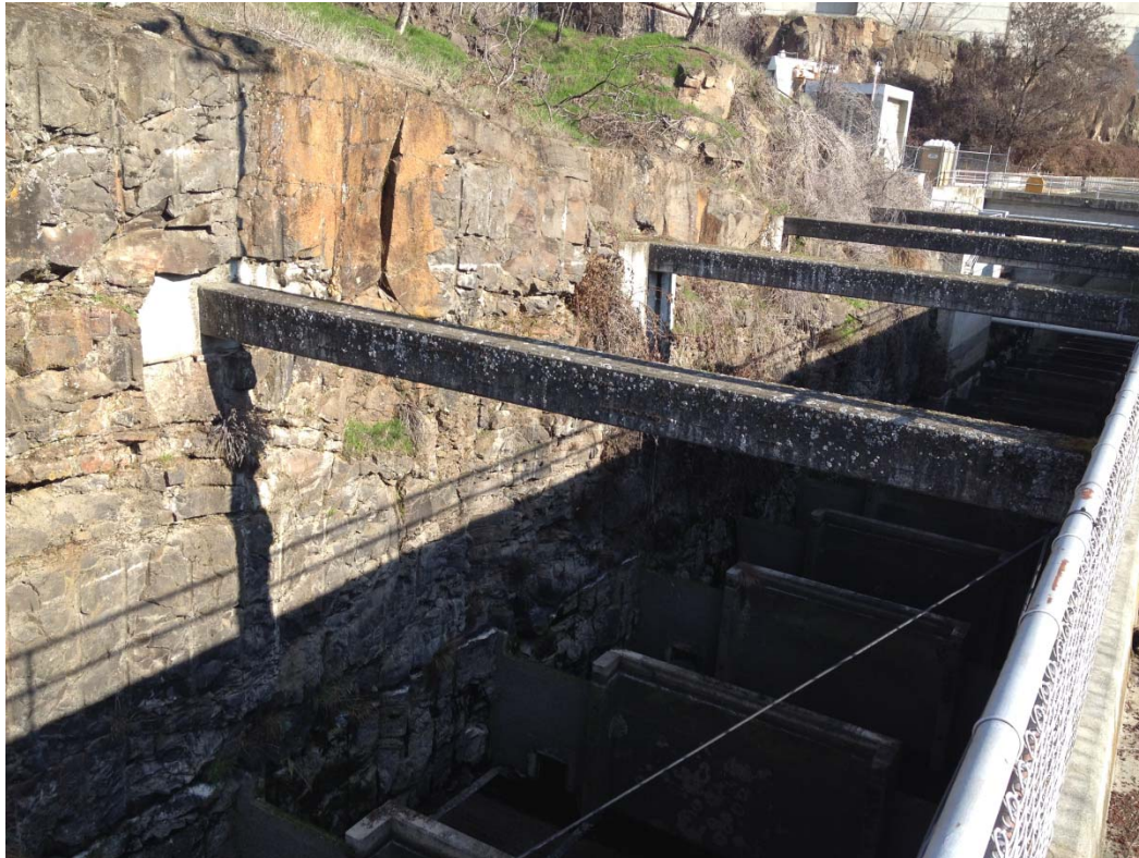
Figure 4 – Photograph looking north-northeast towards section of fish ladder between weirs No. 77 and 92. Note concrete struts supporting wall to the right of the photo.
