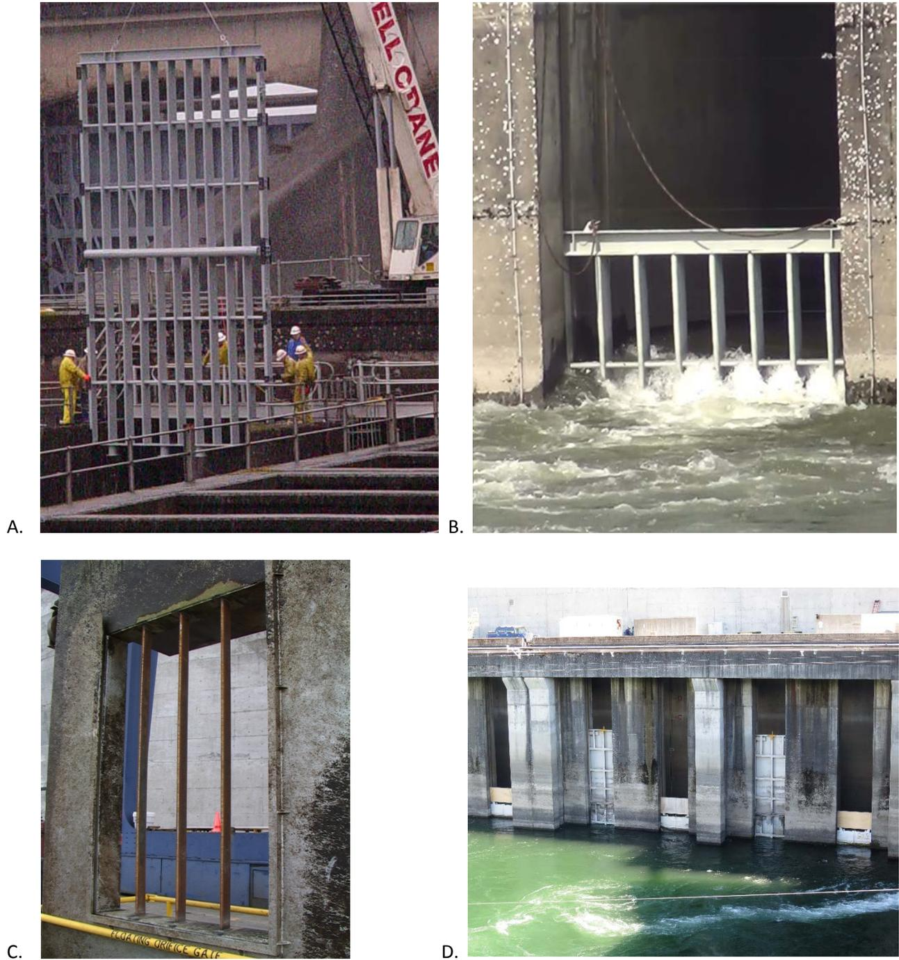
Figure 14. Sea lion exclusion device (SLED) at Bonneville Dam fishway entrance (A) (Tackley et al. 2008) and installed (B) (photo by Bjorn van der Leeuw, USACE FFU), floating orifice gate (FOG) (C) (unknown source), and sea lion incursion barriers on top of FOGs (D) (photo by Patricia Madson, USACE FFU).
