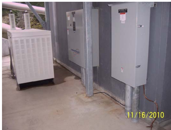
Figure 13 – Emergency Generator
