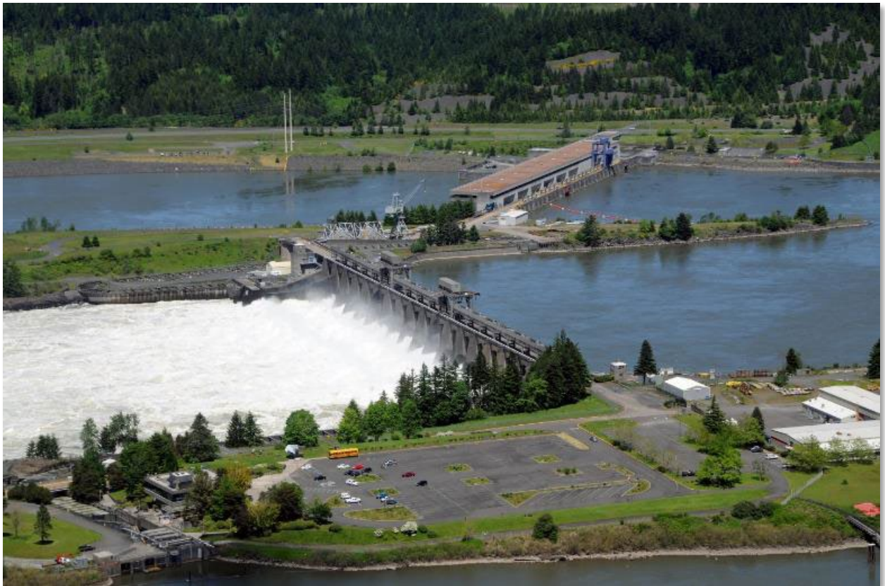
Spill at Bonneville Dam
